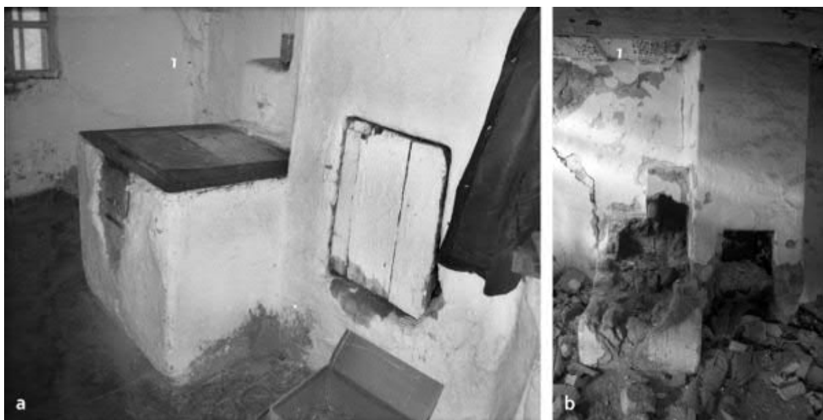
Fig. 6: Koromľa (Slovakia, Sobrance District), Nr. 114, walled stove and chimney in the kitchen: a – State in 1997 (photo by V. Sinčáková); b – State in 2018 (photo by M. Volovár).
